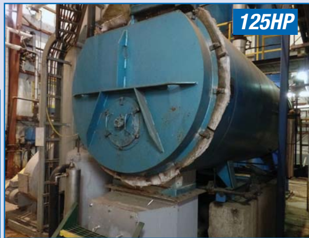
CLEAVER BROOKS STEAM BOILER
