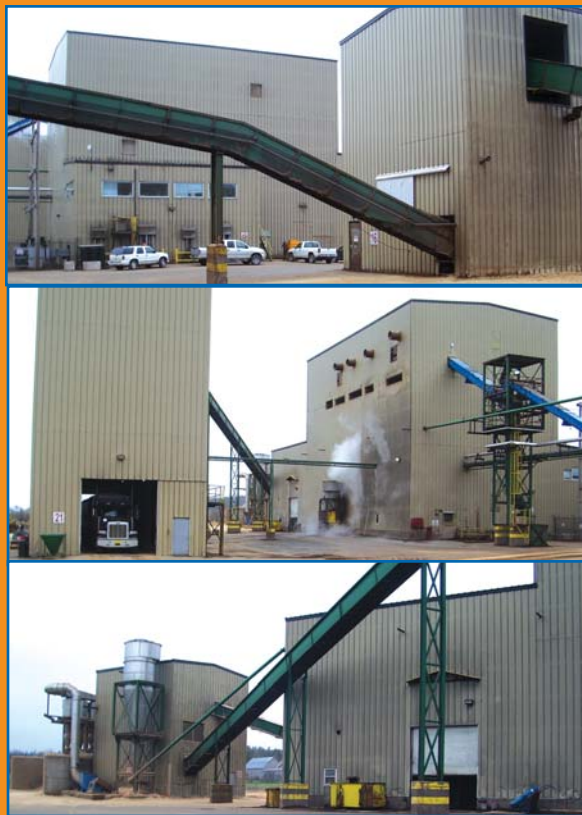
PARTIAL VIEW OF BUILDINGS, TRANSFORMERS, TEC CABLE & ELECTRICAL
