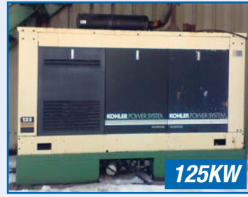
KOHLER 125 DIESEL GENERATOR
